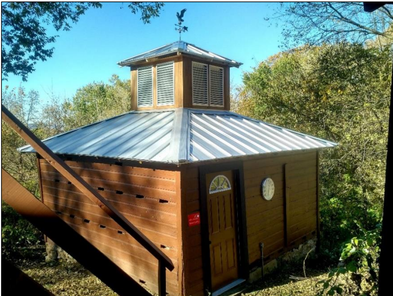
Thrive! Center Beehouse, Renovated/Restored, 1885 Era
